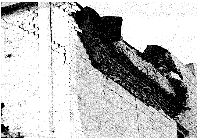
Fig. 9. Out-of-plane failure of exterior wythe of multi-wythe walls having poor-quality collar joint, near 4th Street and Santa Monica Boulevard, Santa Monica.
