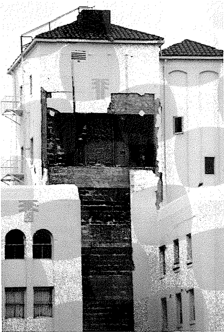
Fig. 6. Parapet failure, Henshey's Men Clothing Shop, Santa Monica Boulevard, Santa Monica.
