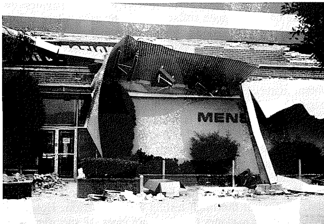
Fig. 6. Parapet failure, Henshey's Men Clothing Shop, Santa Monica Boulevard, Santa Monica.
