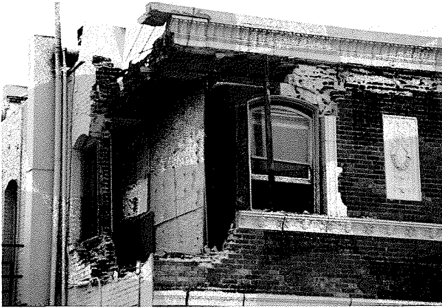
Fig. 22. Severe corner damage in retrofitted building: collapsed corner wall L-shaped in plan, Hollywood Boulevard, Hollywood.
