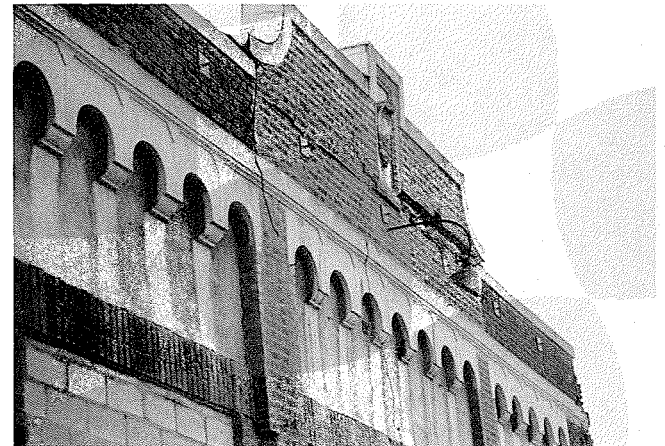
Fig. 20. Out-of-plane failure and near collapse of the central taller portion of a parapet, due to an incomplete retrofit, Washington Street, Culver City.
