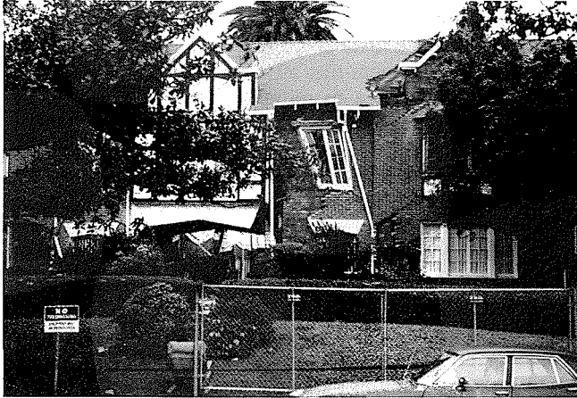
Fig. 1. In-plane damage to nonstructural masonry veneer, Ye Old San Vicente Apartments, Santa Monica.
