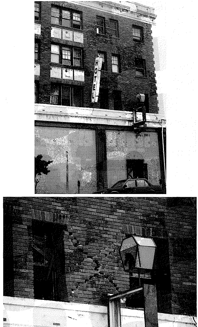
Fig. 27. Damaged retrofitted Staton Hotel, Western Avenue, Hollywood: (a) global view; (b) severe in-plane X-cracking of piers.
