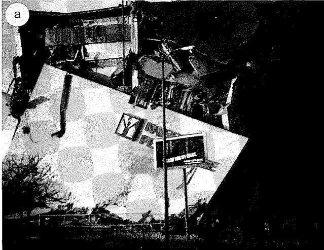
Fig. 34. Collapse of the Northridge Kaiser Permanente Medical Center, a five-story reinforced concrete building having solid stiff reinforced brick masonry wall spanning the short direction: (a) global view of collapse in the north-south direction; (b) closeup view of reinforcement details of end walls.
