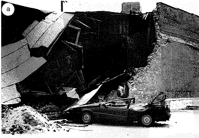
Fig. 18. Out-of-plane wall failure due to unbraced ceilings battering the walls, and inadequate anchorage from intermediate braces at ceiling level, for retrofitted building on Lankershim Boulevard, in North Hollywood: (a) global view of failed wall; (b) closeup view of roof anchorage and wall construction.
