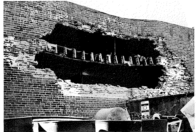
Fig. 19. Out-of-plane wall failure due to ineffective intermediate braces and battering action of unbraced ceilings, for retrofitted building located on Washington Street, Culver City.
