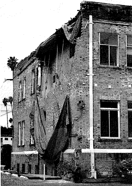
Fig. 16. Out-of-plane failure of top-story two-wythe brick unreinforced masonry wall and one-wythe veneer of a retrofitted building in Hollywood, due to excessive height-to-width ratio.
